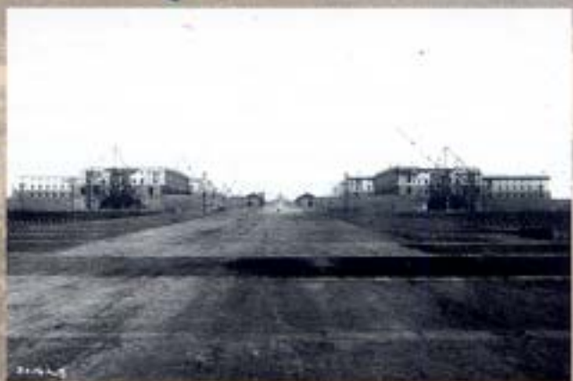
North & South Block under construction.
